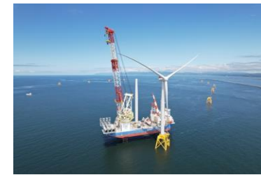
Turbine Generator Installation
